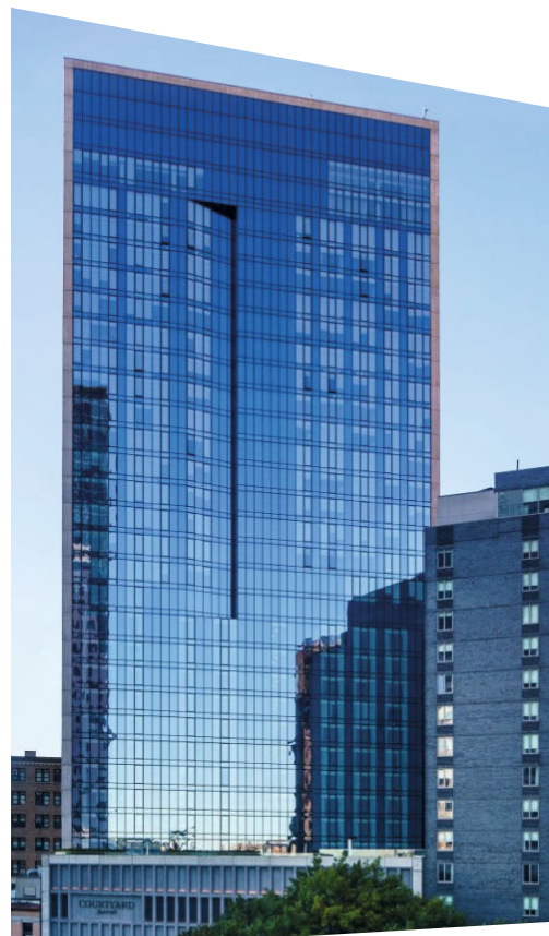
(LIC Mariott) 29-07 Queens Plaza North, NYC, NY Handel Architects LLP
